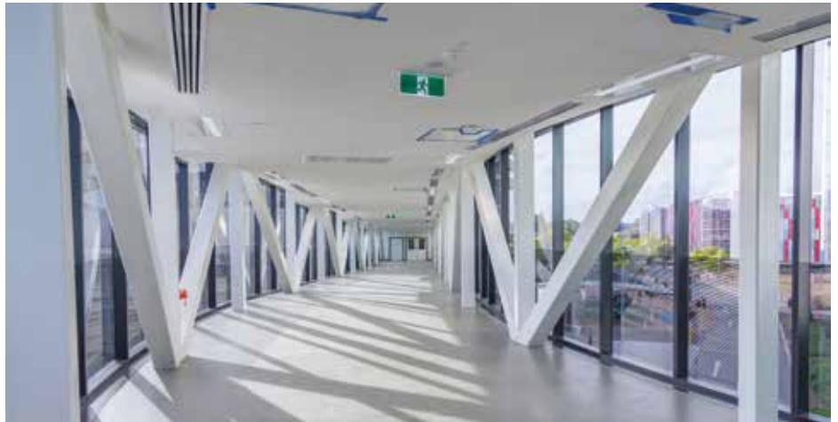
PCH link bridge: Over 140 tonnes of structural steel was used to construct the bridge over Hospital Avenue
